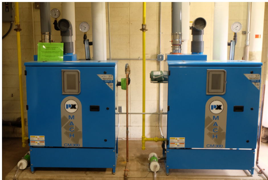
HVAC upgrades at Crescent High School included two Paterson-Kelley condensing boilers.
