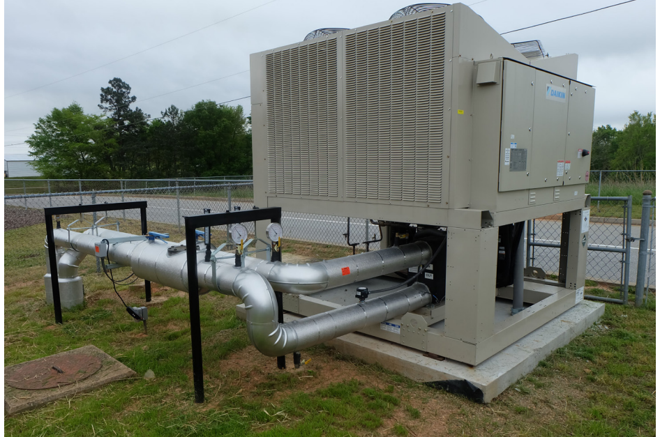
To save water, ABM replaced water-cooled chillers with air-cooled chillers, like this Daikin air-cooled chiller at Starr Elementary.
