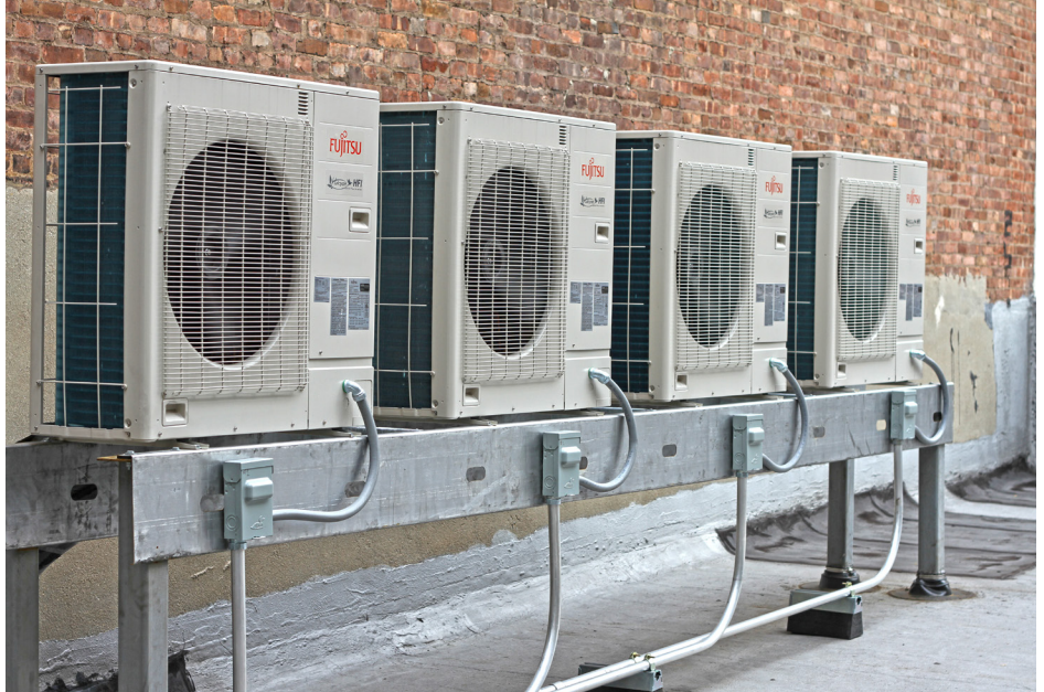
Custom steel framework was erected to mount the units several feet above the flat roof.
