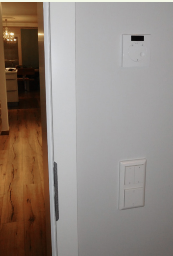
Left: Temperature control via Afriso wall thermostat. Roller shutter and lighting control via OPUS® switch design Inform.
