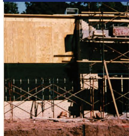
PHOTO 5 Old School. Apparently, a point missed by folks is that we installed asphalt impregnated felt, Type D-coated building papers and building wraps by nailing and stapling them, and then we nailed and screwed cladding systems through them and did nothing special at the resulting penetrations and the world did not come to an end.
