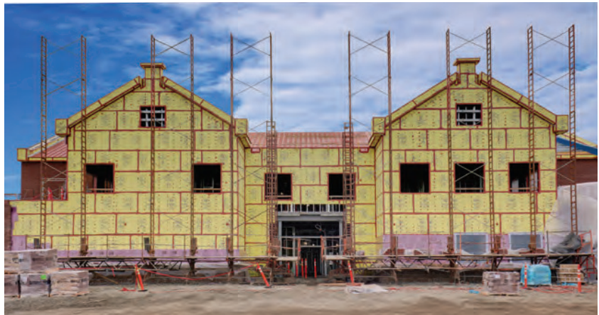
PHOTO 5 Old School. Apparently, a point missed by folks is that we installed asphalt impregnated felt, Type D-coated building papers and building wraps by nailing and stapling them, and then we nailed and screwed cladding systems through them and did nothing special at the resulting penetrations and the world did not come to an end.
