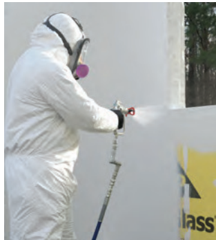
PHOTO 1 (TOP LEFT) New Systems. The trend is to sheet goods covered with spray-applied liquid membranes. Note the word “sheet goods.” PHOTO 2 (TOP RIGHT) More New Systems. Gypsum board sheets covered with trowel applied membrane. PHOTO 3 (BOTTOM) Still More New Systems. Sheet goods with integral water and air control layers.
