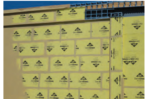
PHOTO 1 (TOP LEFT) New Systems. The trend is to sheet goods covered with spray-applied liquid membranes. Note the word “sheet goods.” PHOTO 2 (TOP RIGHT) More New Systems. Gypsum board sheets covered with trowel applied membrane. PHOTO 3 (BOTTOM) Still More New Systems. Sheet goods with integral water and air control layers.
