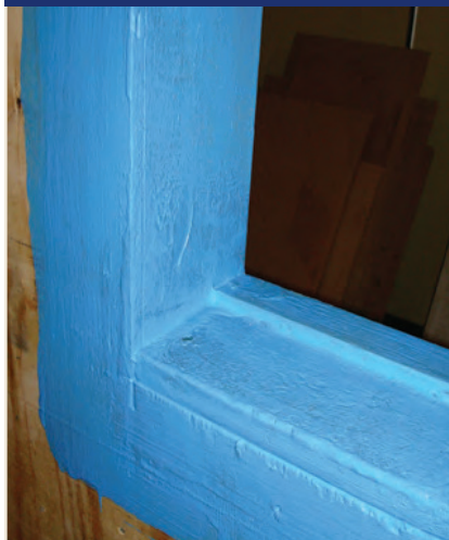
PHOTO 4 Window Opening. Lots of joints and inside and outside corners. How we deal with the joints and the inside and outside corners is the trick. Note the “fillet” sealant in the “end dam” and “back dam” under the liquid-applied membrane.
